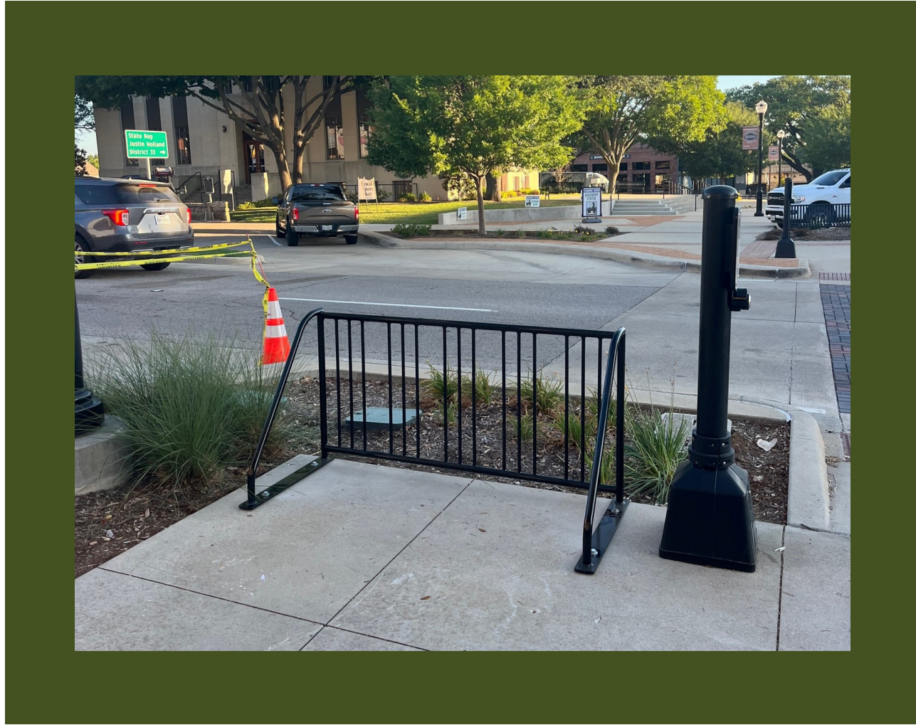
SAN JACINTO PLAZA BIKE RACK INSTALL
